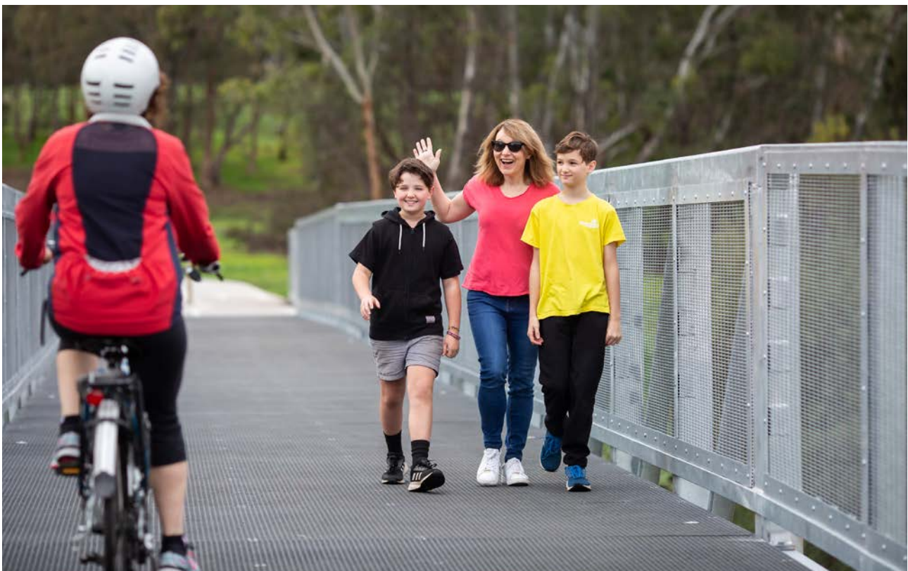
Rathcown Road Bridge, Reservoir
