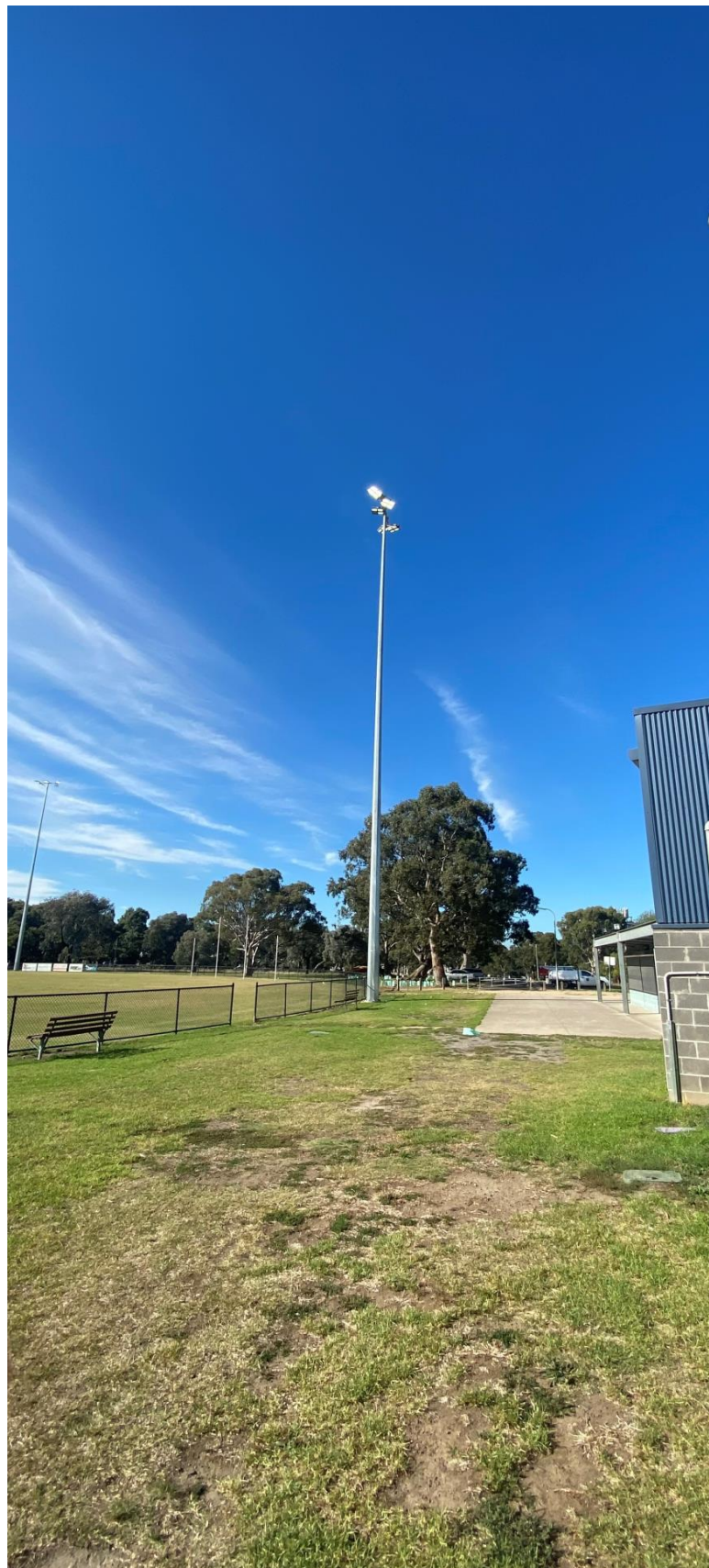
Attachment 1 – Photograph showing existing sports oval light
