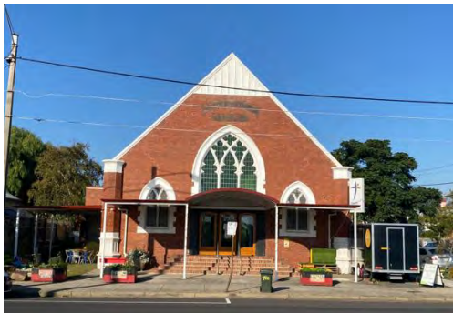
Thornbury Church of Christ, 390—398 St Georges Road, Thornbury, Source: Extent Heritage Pty Ltd, 2024.
