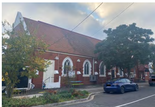
View from Smith Street of south elevation of Thornbury Church of Christ.
