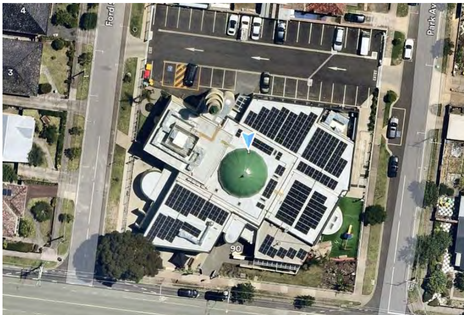
Figure 7. 2022 aerial of the Omar Bin El Khattam Mosque, showing enlarged footprint. Source: Nearmap, 2022.
