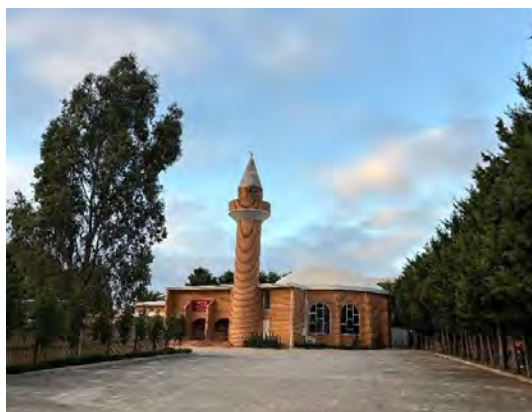
Photograph of 111 Blake Street, Reservoir. Source: Extent Heritage Pty Ltd, 2024.
