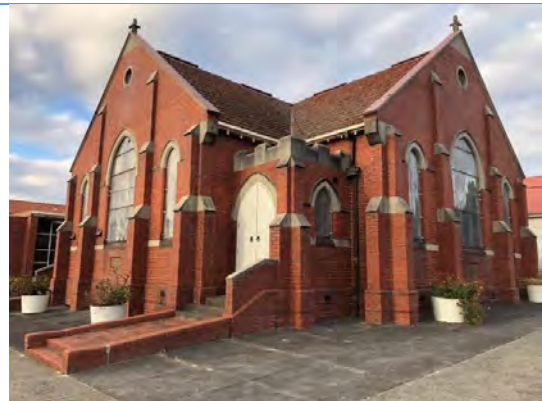
Entrance to the Methodist Church, looking northeast, showing the western and southern gables. Source: Extent Heritage Pty Ltd, 2024.
