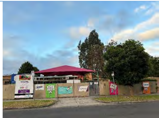
View of the Reservoir Albanian Mosque from Blake Street, where views of the building have been obscured by the Kindergarten building in front.
