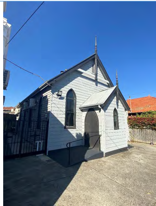
Oblique view of the original timber Methodist Church (source: Extent Heritage Pty Ltd, 2024).
