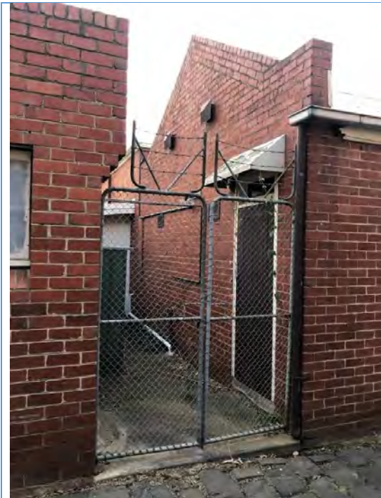
Oblique overview of the Kindergarten gable looking northwest. Source: Extent Heritage Pty Ltd, 2024.
