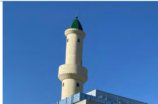
Figure 15. Detail view of minaret. Source: Extent Heritage Pty Ltd, 2024.
