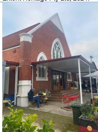
View from north showing column on the north corner surmounted with crenulated finishes. Source: Extent Heritage Pty Ltd.
