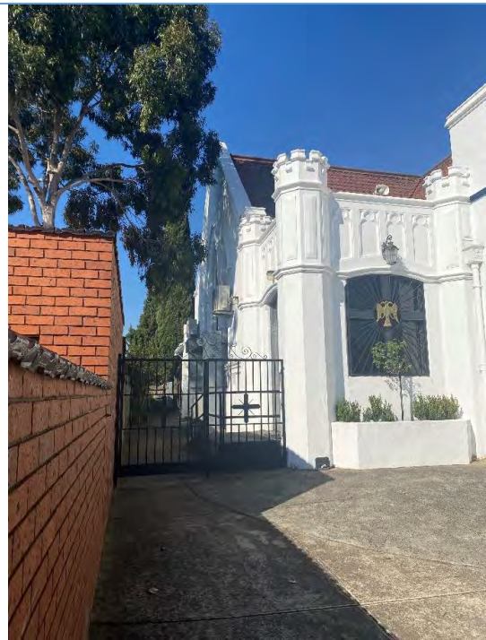
Detail view of the northern boundary of the site including the northern transept of the Greek Orthodox Church (source: Extent Heritage Pty Ltd, 2024).
