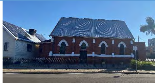
Eastern elevation of the Church. Source: Extent Heritage Pty Ltd 2024.
