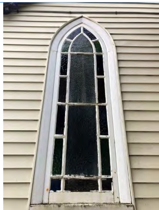
Western lancet window on the Church Hall façade. Source: Extent Heritage Pty Ltd, 2024.
