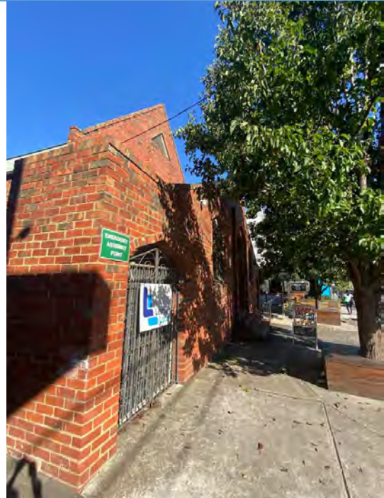
Detail view of wrought iron gate and doorway to the front façade. Source: Extent Heritage Pty Ltd.
