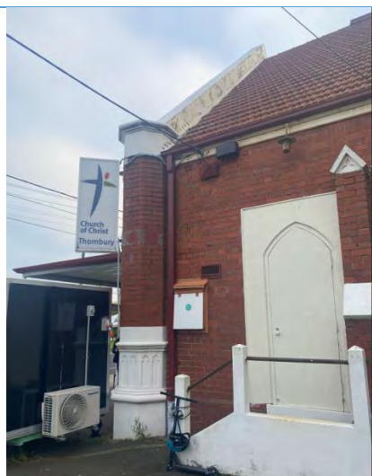
View from south showing column on the south corner surmounted with crenulated finishes. Source: Extent Heritage Pty Ltd.
