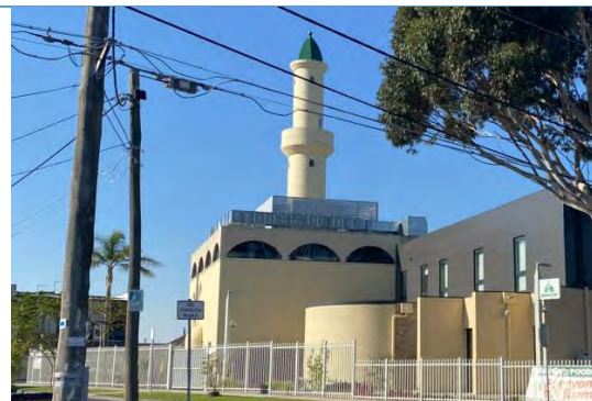
Figure 11. Oblique overview of western elevation from Ford Street. Source: Extent Heritage Pty Ltd, 2024.
