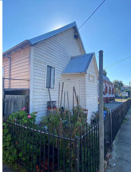
Oblique view of the Church Hall looking north. Source: Extent Heritage Pty Ltd 2024.
