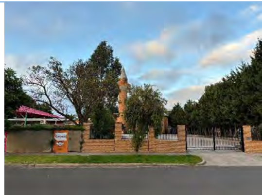
View of the Reservoir Albanian Mosque from across Blake Street, showing minaret. Source: Extent Heritage Pty Ltd. 2024.
