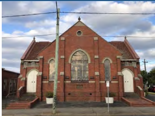
Overview of the Former Croxton Methodist Church façade, looking east. Source: Extent Heritage Pty Ltd, 2024.
