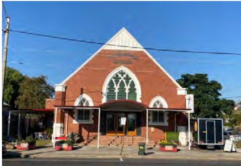
Thornbury Church of Christ, 390—398 St Georges Road, Thornbury, Source: Extent Heritage Pty Ltd, 2024.
