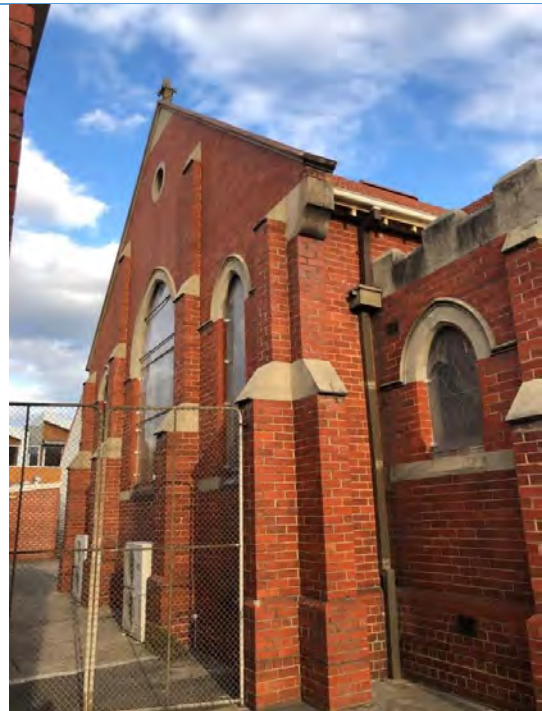
Oblique view of the northern gable. Source: Extent Heritage Pty Ltd, 2024.
