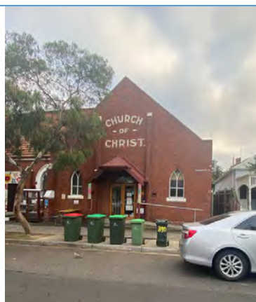
View from Smith Street (south) of façade of original Thornbury Church of Christ constructed c 1922.
