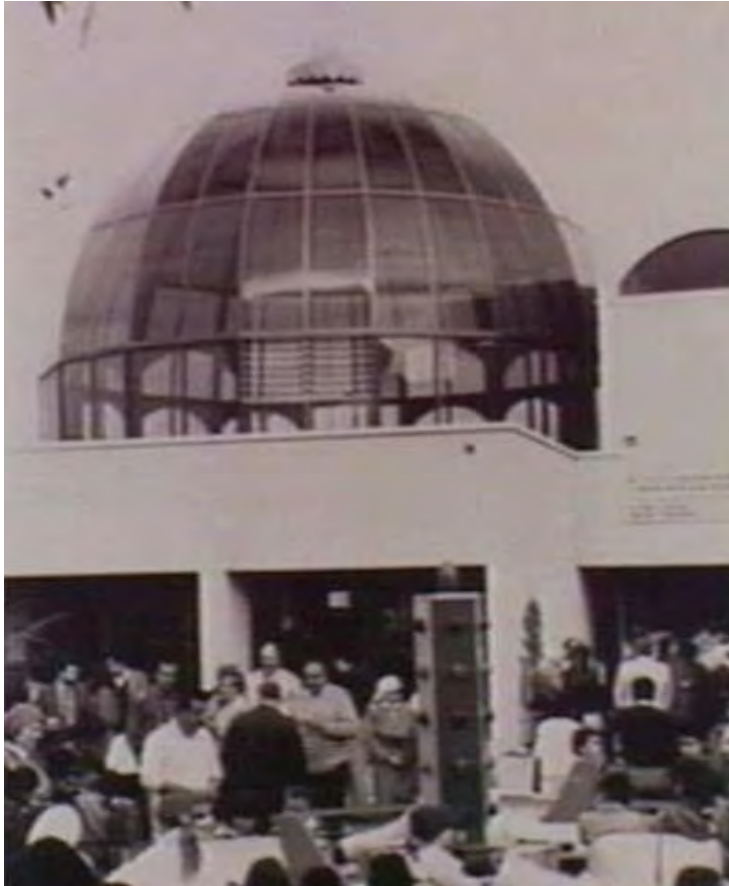
Figure 5. 1987 photograph of glazed dome addition. Source: Hage, F E.. 1988. The celebration of Id El Fitr at Preston Mosque, 1987. Digitised photograph. In collection: Fouad El Hage Photographs. Accession No : H92.250/1338
