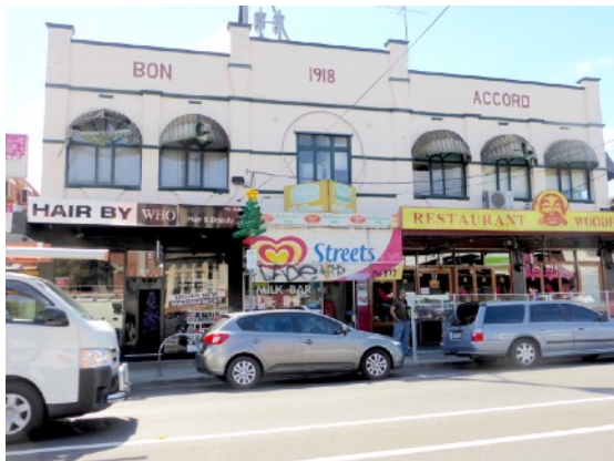
Figure D1. View illustrating one of the larger and very wide two storey heritage places divided into narrow shop fronts which is reflected in the design of the first floor rendered walls. The first floor is divided into vertical bays with pilasters emphasised by a large round arched window between them, the high parapet is divided into three bays which is emphasised by the broken skyline. Thin horizontal lines balance the verticality of the narrow bays.
