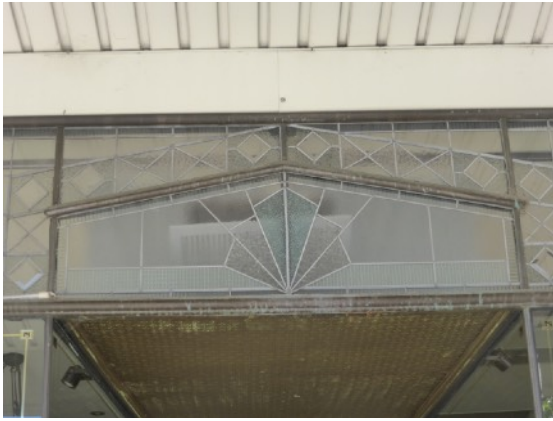
Figure D6. The top lights of this shop window are in the Art Deco style and the ceiling of the ingo is pressed metal.
