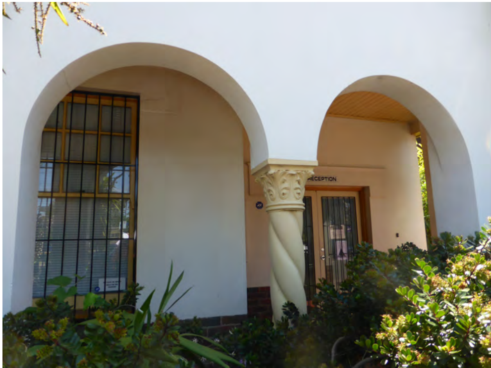
Figure D3. Elaborate twisted decorated column with acanthus leaf capital, rendered walls above the dado of clinker bricks, rectangular timber windows with nine lights over one, and timber doors and timber lined ceiling.
