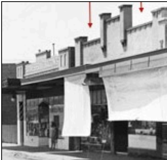
FigureD2. Detail of Figure H4. Railway Place showing the street front of 5 and 5a looking from Rathmines Street towards Gillies Street (estimated c.1928-greater than c.1946). Photographer unknown, n.d., Source: Railway Negatives Public Record Office Victoria VPRS12800/P0003/44 (reproduced with permission)
