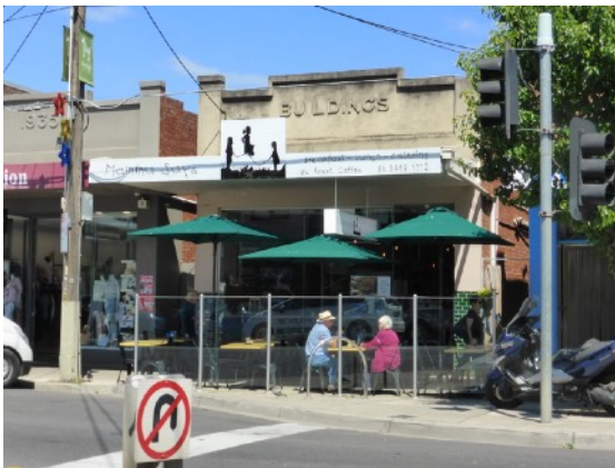
Figure D3. Typical example of a modest single storey unpainted red brick historic place with a cantilevered verandah, and intact unpainted rendered parapet with broken skyline, formed by pilasters with simple 'capitals' and the name of the original building complex in relief, '1935 BUILDINGS' from the Inter-war era of development. It is likely that this was built as a set of three.
