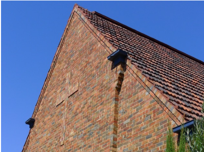
Figure D2. Understated detailing using clinker bricks to create a finely articulated surface including two lines of brick ( one headers and one stretchers) following the angle of the gable end, a thin corbelled projection, and a cross made entirely of bricks set vertically. Overall the north facade has a minimalist and modernist approach to the design.
