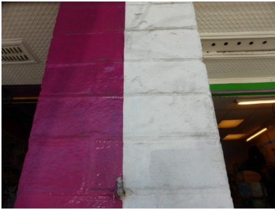
Figure D11. Several shop fronts have tuck pointed brick work. Now overpainted, the delicate and skilled craft of tuck pointing can be revealed on the historic shopfronts by chemically removing the paint.
