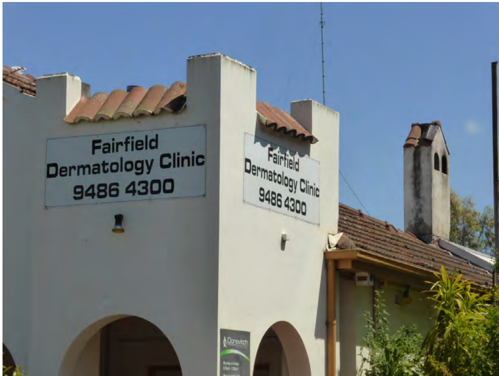
Figure D2. Distinctive parapeted entry porch with Spanish tiles, and gabled chimney top with round arched openings and Spanish tiles.
