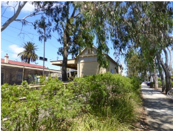
Figure D16. View along Wingrove Street from Station Street, of the north and south station buildings, set in the historically spacious railway reserve with one of the two palm trees on the south side, visible above the roof
