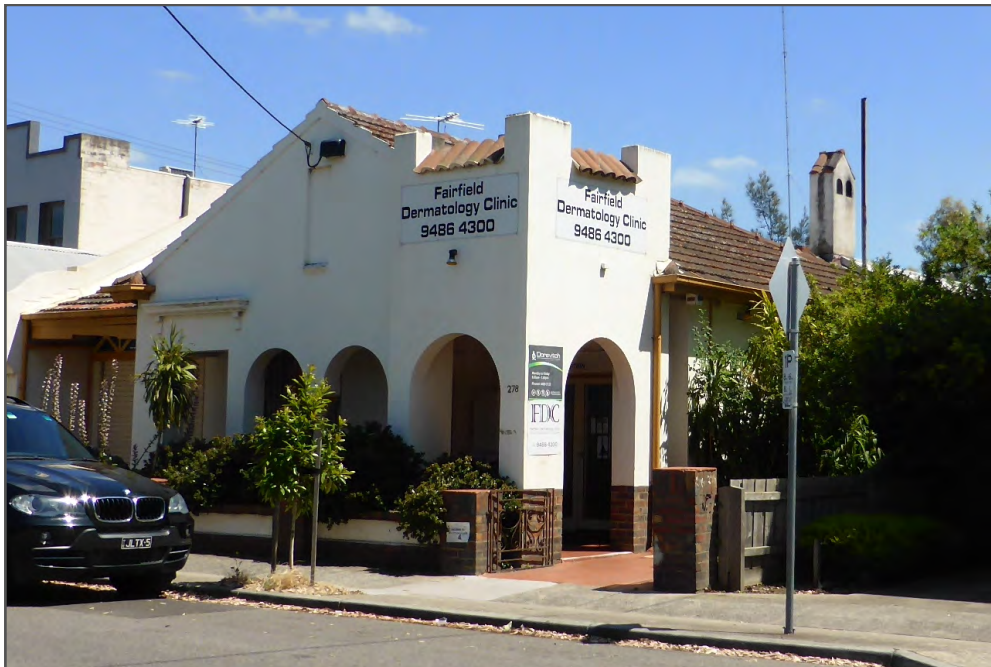
Figure D1. View showing the Spanish Mission style features of rendered walls above sill height, clinker brick dado, round arched loggia, Spanish tiles, gable end, distinctive surgery entry parapet, gabled chimney top and ledge moulding over the residence entry.
