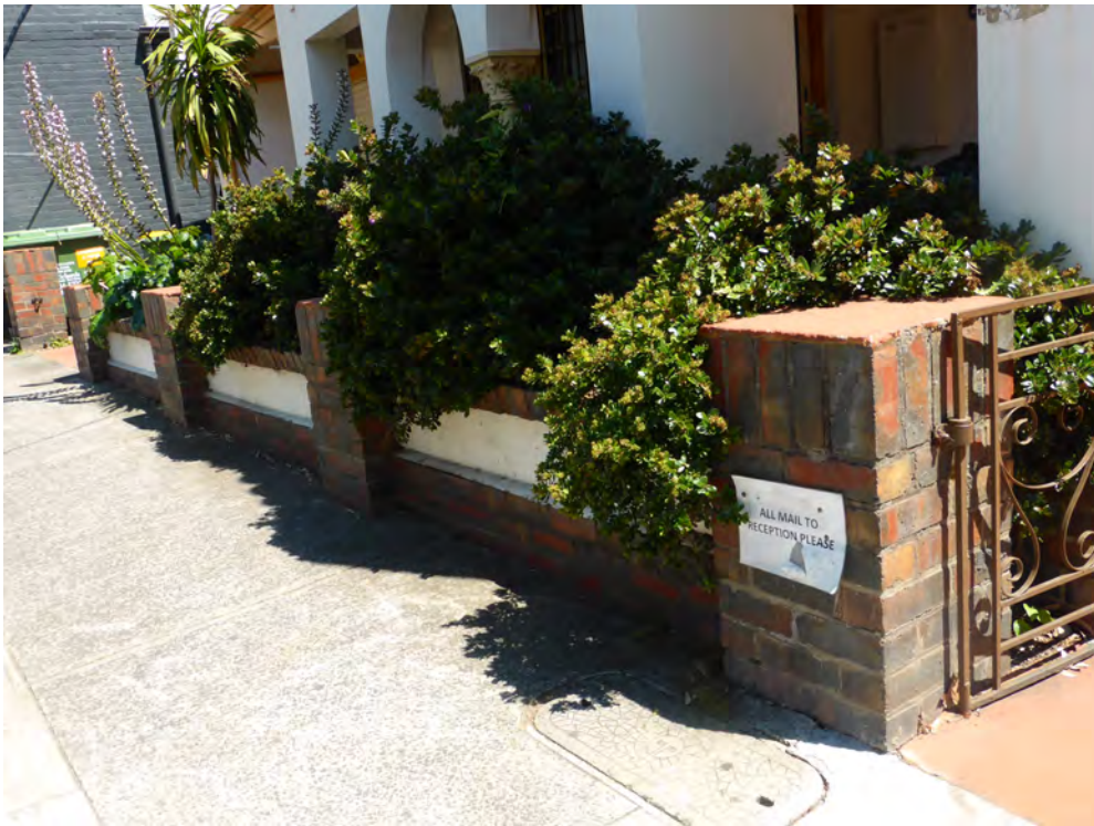
Figure D4. The low fence has been designed to match materials and features of the building, showing rendered panels between clinker brick plinth and angled clinker brick headers, supported by clinker brick piers.
