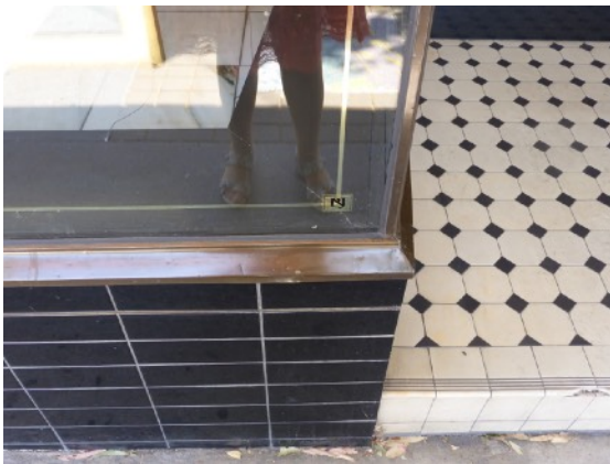
Figure D7. Several shop front windows have retained their Inter-war thin copper/brass metal window frames, deep stall boards of glazed tiles, ingoes with encaustic tiled floor patterns.
