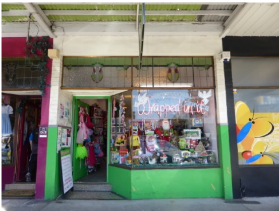
Figures D9 and 10. Several shop fronts have historic lead light top lights in the colours and patterns of the Art Nouveau style.
