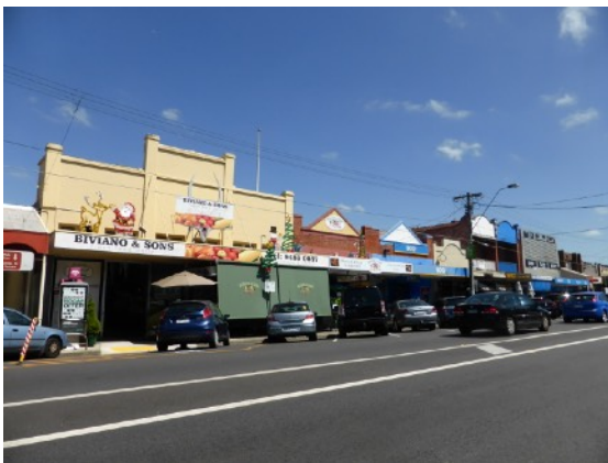
Figure D4. The streetscape view illustrates the variety in heights of the one and two storey heritage places and skylines using similar materials and features on the buildings: rendered parapet using pilasters to divide them into narrow bays as well as pilasters (in brick and/or render) at each end of each property.
