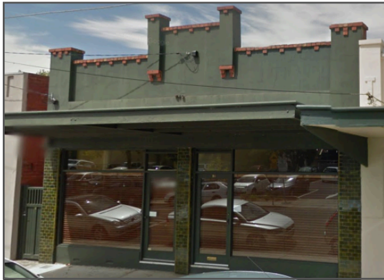
Figure D1. View showing the Inter-War Art Deco style features of rendered and stepped parapet with stylised low relief contrasting red brick 'cornice' with dentils below. The parapet is divided into three bays by rendered pilasters, with the central bay surmounted by a raised parapet. The ground floor shop fronts have been altered. Note the gate on the east side, which provided access to the residence at the rear. Source: Google street view.
