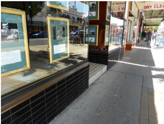
Figure D8. Pedestrian level view of the human scale of the historic shop fronts which are divided into narrow bays and deep ingoes, and fine decorative details.
