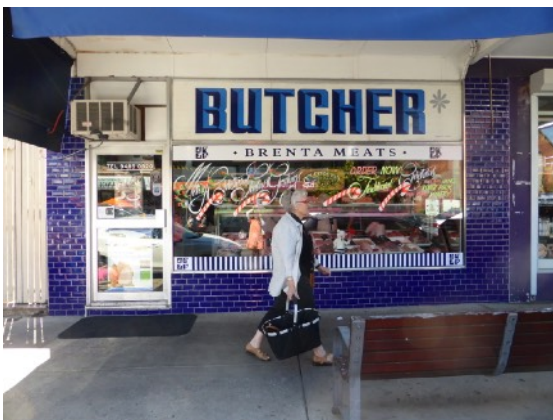
Figure D5. The butcher shop illustrates an Inter-war shop front with a large window and highlight windows above it, surrounded by a thin metal window frames and glazed tiles on the piers and deep stall board below the window frame. ( The door is more recent.)
