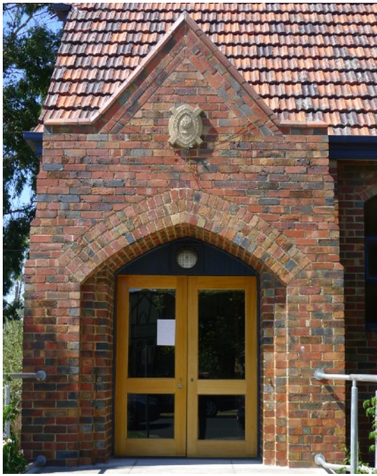
Figure D4. The traditionalist Gothic design of the entry porch, facing Gillies St. The pointed arches are emphasised by the three rows of soldier headers over the entry porch, and three rows of stretchers following the line of the gable end. Vertical 'engaged piers' support the entry arch and an unpainted crest in-relief of the Presbyterian Church of Australia is visible, in the gable end.
