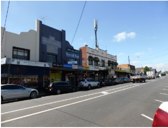
Figure D2. Distinctive parapets of two historic places illustrate the variations in design of the broken skyline and the more human scale achieved by the division of these large wide buildings into narrower bays.
