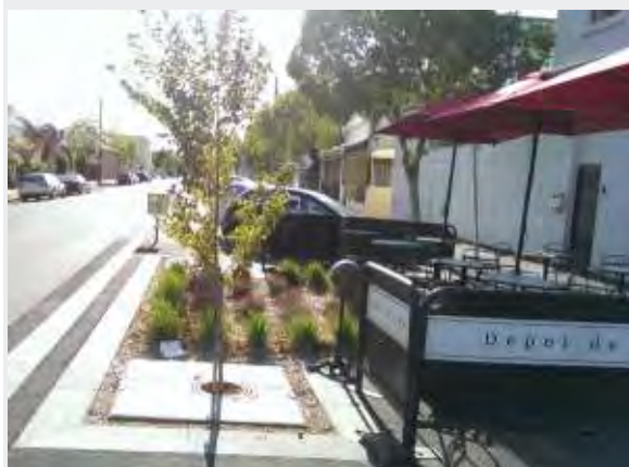
Rathdowne Street Carlton - Kerb Outstands Provide Transition Between Commercial and Neighbourhood Streets Allowing Additional Planting and Activation Image: Outlines Landscape Architecture
