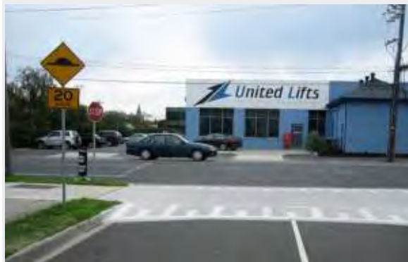
Raised Crossings Enhance Pedestrian Accessibility and Priority Image: bicyclenetwork.com.au
