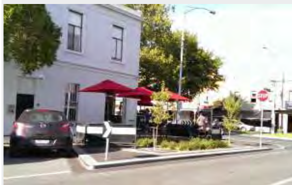
Rathdown Street Carlton - Kerb Outstands Reduce Crossing Distances and Provide Greening Opportunities Image: Outlines Landscape Architecture
