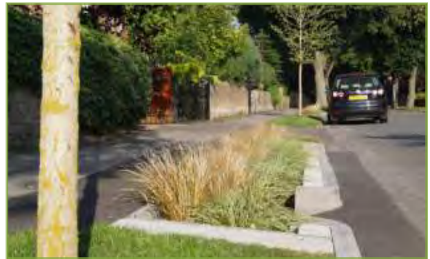
The Environment - Retrofit Rain Garden Project Assist in Stormwater Management Image: isusdrain.org
