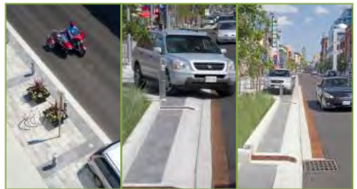
King Street Kitchener - Removable Bollards and Sloping Kerbs Enable Flexible Use of Public Space Images: IBI Group via worldlandscapearchitect.com
