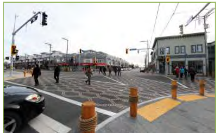
Robson Street Vancouver - Scramble Phase Crossing Pilot Project With Clearly Defined Crossing Zones Image: binnie.com
