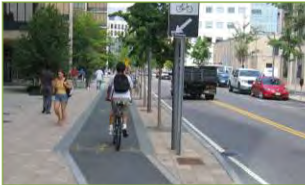
Back of Kerb Bicycle Lane - Provides Unified Street with Integrated Bicycle Infrastructure Image: www.sf-planning.org
