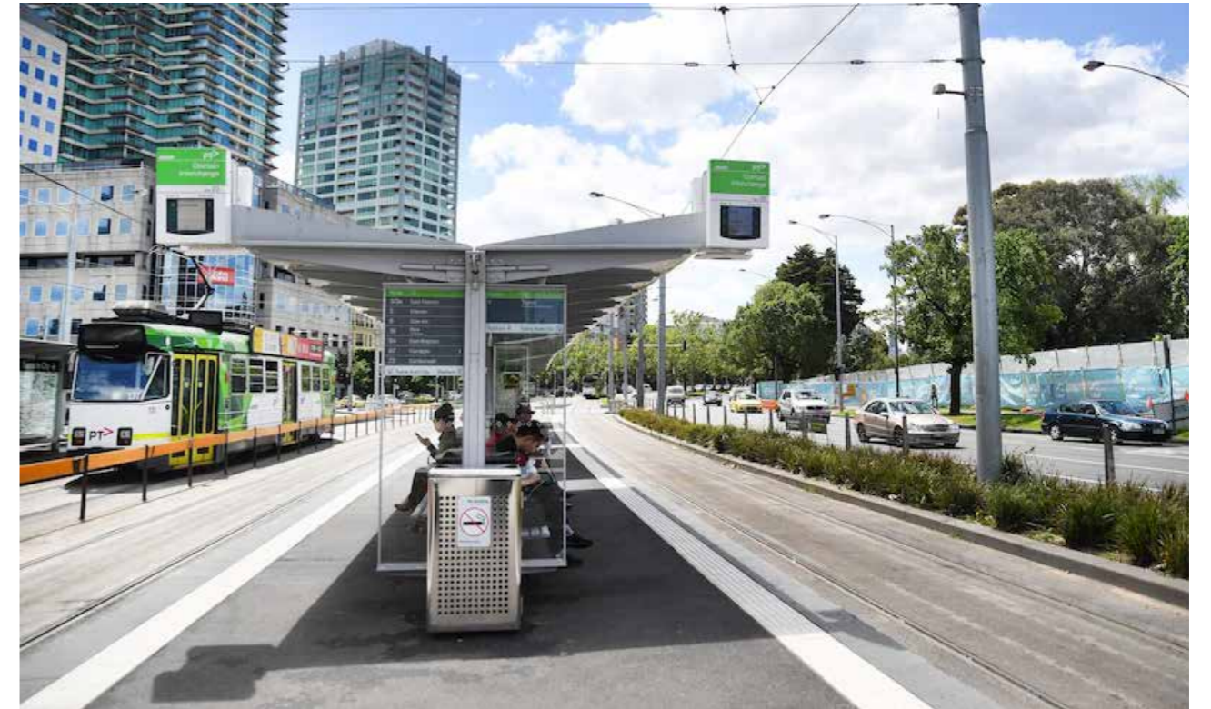
Example of a centre island tram stop at Domain Interchange (now closed due to construction of ANZAC Station) Source: ABC News
