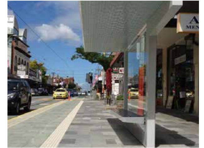
Safe and accessible tram platforms are vital and must meet DDA accessibility standards and use the principles of Universal Design.
