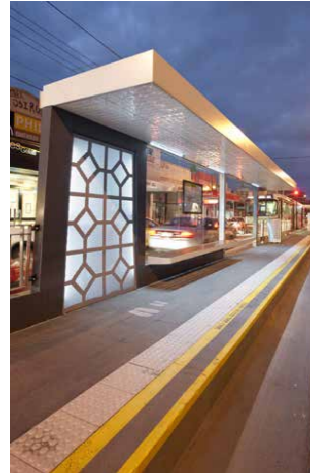
Lighting is provided at all tram stops, avoiding harsh overhead white light where possible.
