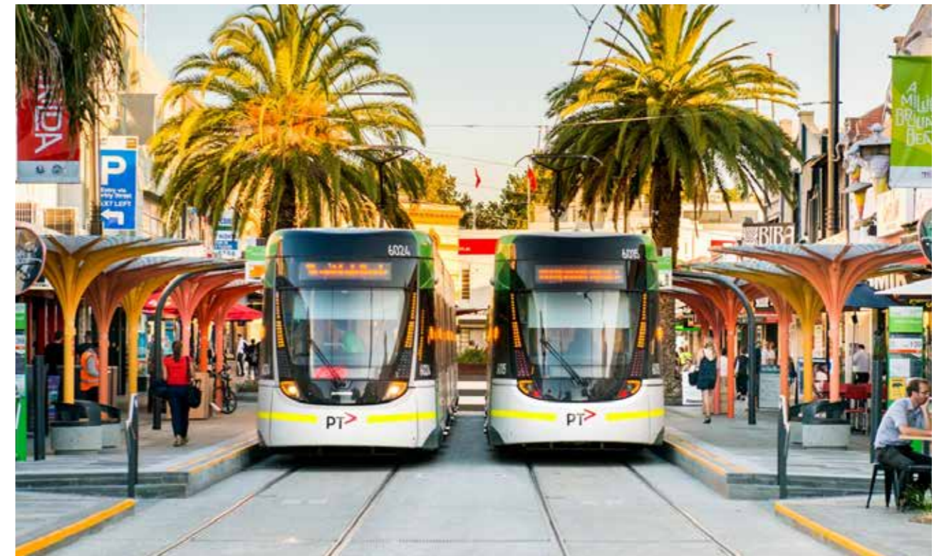
Example of the kerb extension tram stops at Acland Street in St Kilda. Source: Yarra Trams
