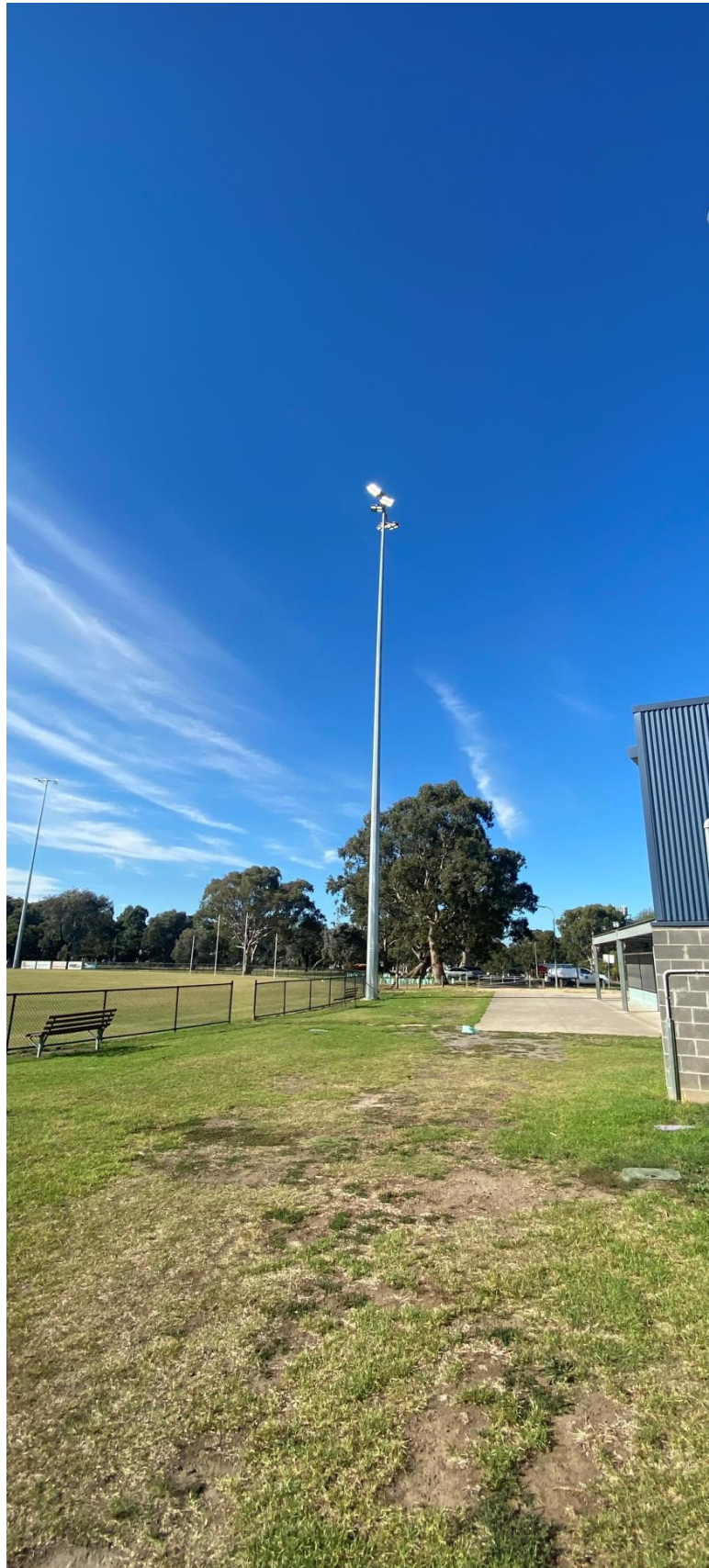
Attachment 1 – Photograph showing existing sports oval light
